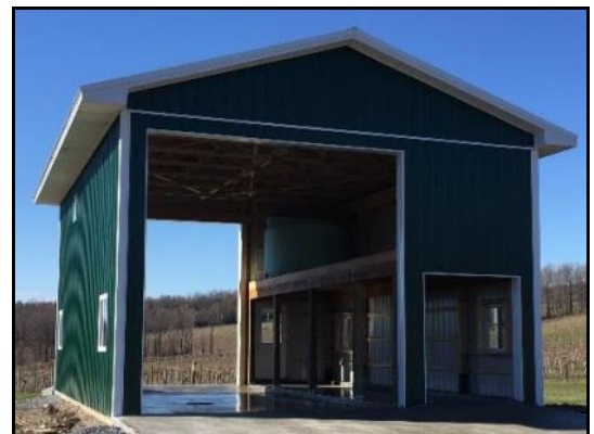
Vineyard chemical mixing station
