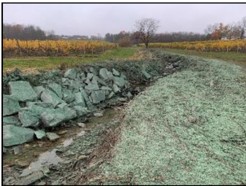
Streambank stabilization
