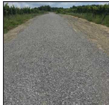
Vineyard laneway erosion control
